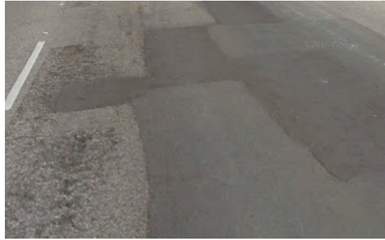
Figure 4 Detail of the end of the section of Highway CE-501
